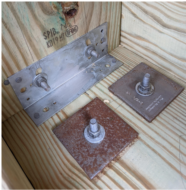
EXAMPLE OF BASE PLATE CONNECTORS
