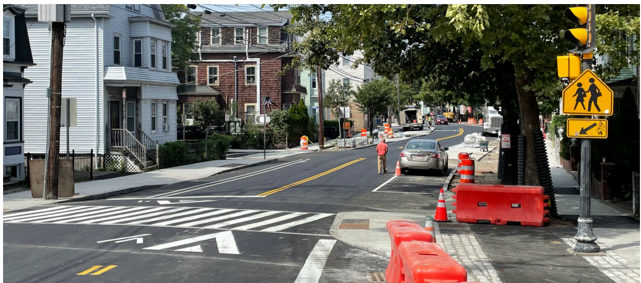
A raised crossing with bulb-out near the Argenziano School in Somerville. (from Streetsblog Mass )
